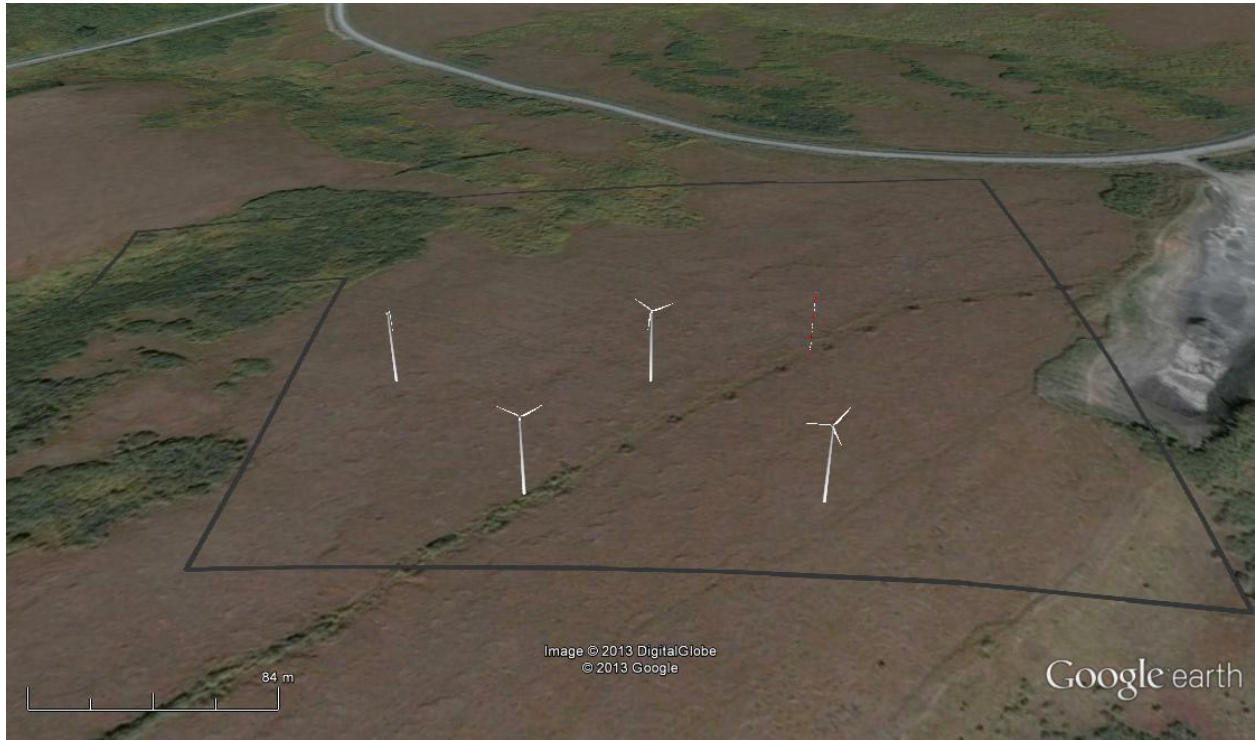
NPS100 ARCTIC turbine layout, view to north
